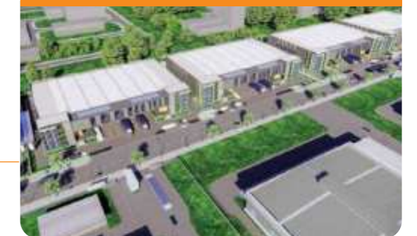
New Ready-Built Factory at Lot 3A Long Hau 3 Industrial Park - Phase 1
