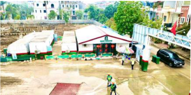
Construction site An Dong, Hai Phong
