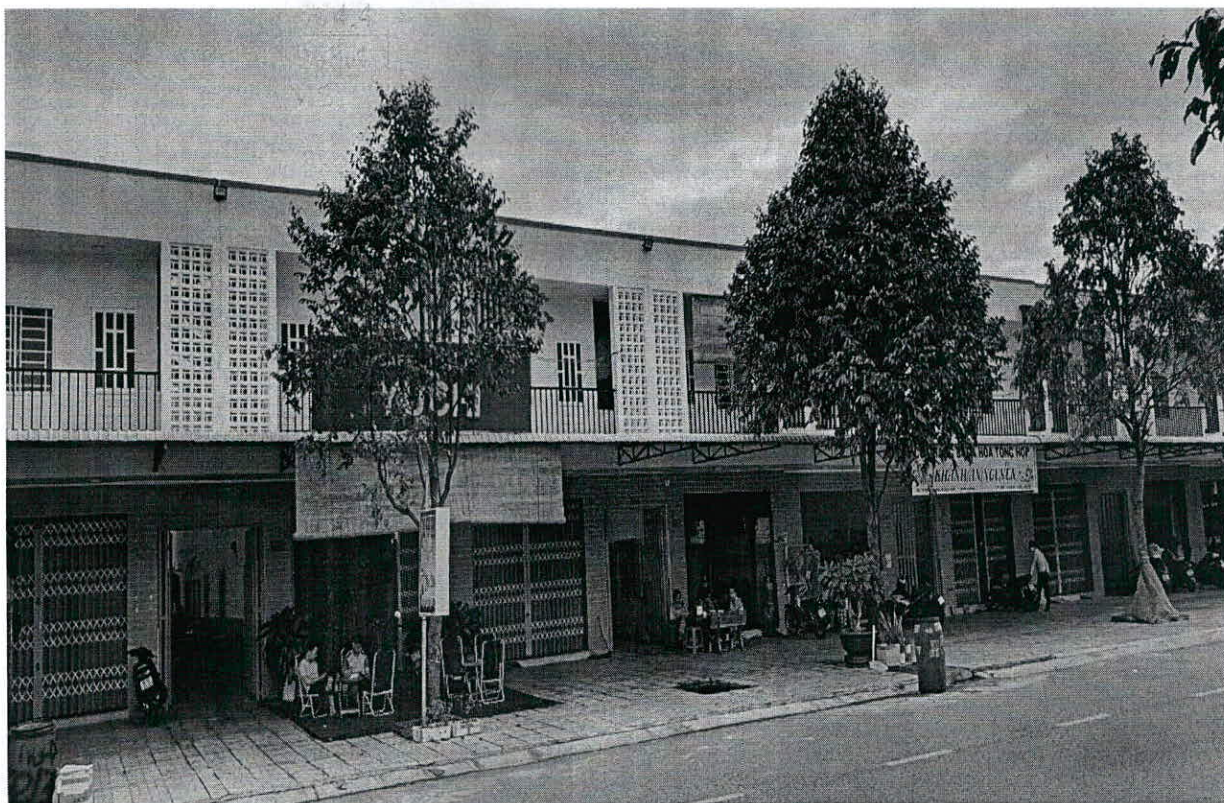
House picture at Plot A51/Bau Bang (Transferred to customers)
